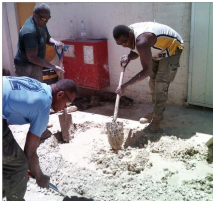
Filling the floor with a concrete base
