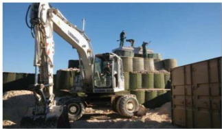
Engineer Corps busy working on the HESCO Wall protection
