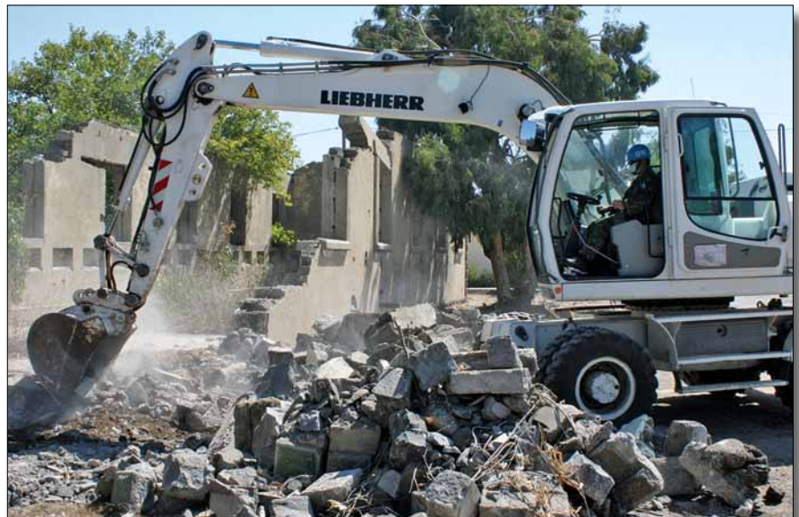
With great skill the operator tears down heavy concrete walls safely
