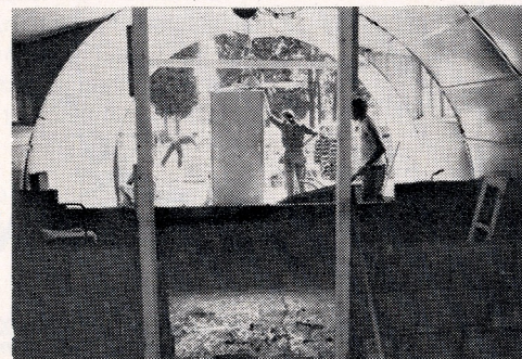
Engineers constructing a Nissan Hut.
