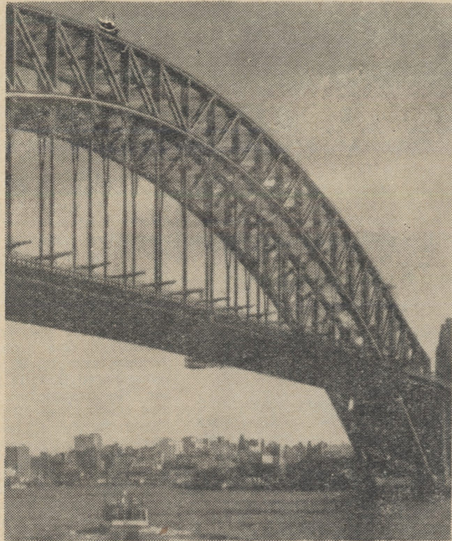
Sydney harbour bridge is a veteran of world fame. Having a span of 1,650 feet it is the world's largest steel arch bridge and carries two electric trains, two footways and an 8 - carriageway road.
