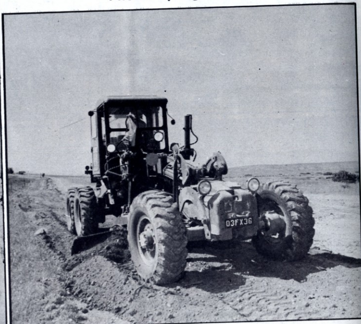
Once the stone is dumped a grader is tasked to level the site in preparation for rolling and compacting.
