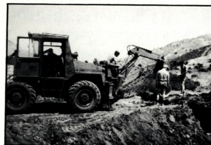
A culvert under construction at DANCON.
