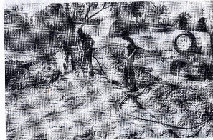
The engineers working on the foundations beneath the pitiless Summer sun.
