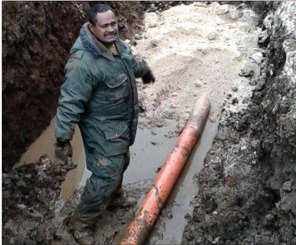
Sgt Buli re-aligning the sewerage pipes in Position 80
