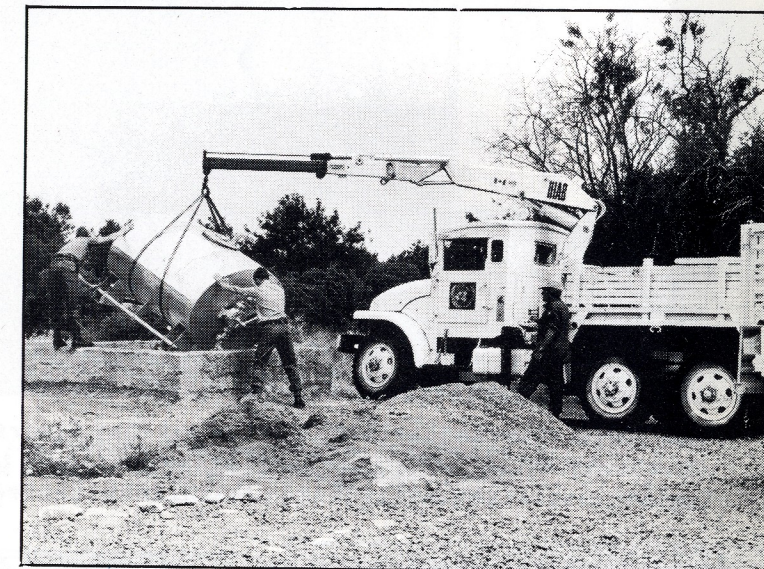
Installation of a bulk AVTUR tank at Limnitis – Sector One
