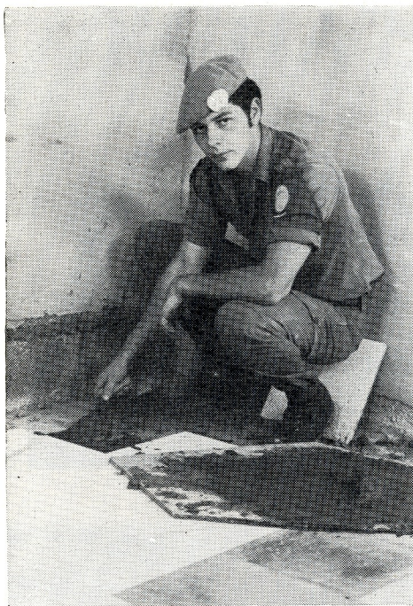
Spr Phil Greatrex laying tiles in a new shower/ablution block in a Sector 2 OP.
